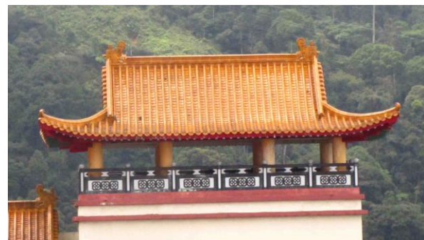
Figure 19: Application of heavy hipped-gabled roof, an influence from Northern Chinese style in a recent Chinese Temple in Pahang
