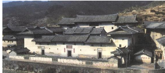
Figure 5: Southern China's architecture- The architecture of commoners' (The three-sectioned gable roof, whitewash walls with no ornamentations, and grey tiles as roof's material are of distinctive characteristics) (Source: Knapp, 2004: 177)
