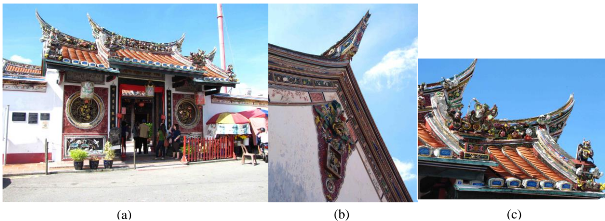
Figure 11: Cheng Hoo Teng Temple, Melaka, 17 th various Southern Chinese influences: a) Overall view-three sections gable roof b) Ornate gable wall c) Ornate raised main ridge and copings
