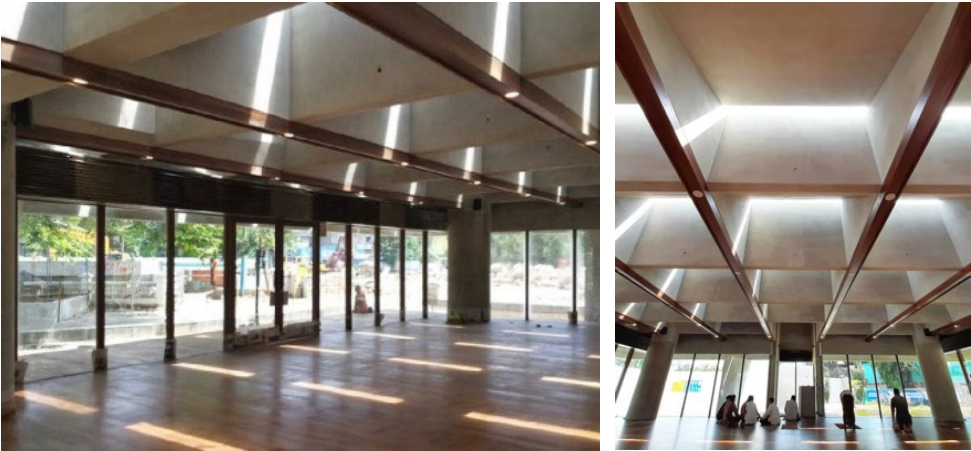
Figure 10. Implementation of natural light inside the prayer room
