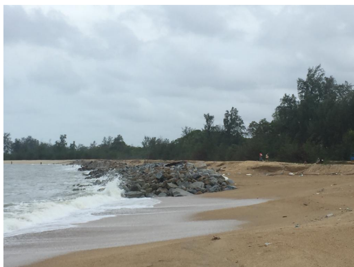
Figure 5: Coastal erosion at Pantai Tok Jembal
