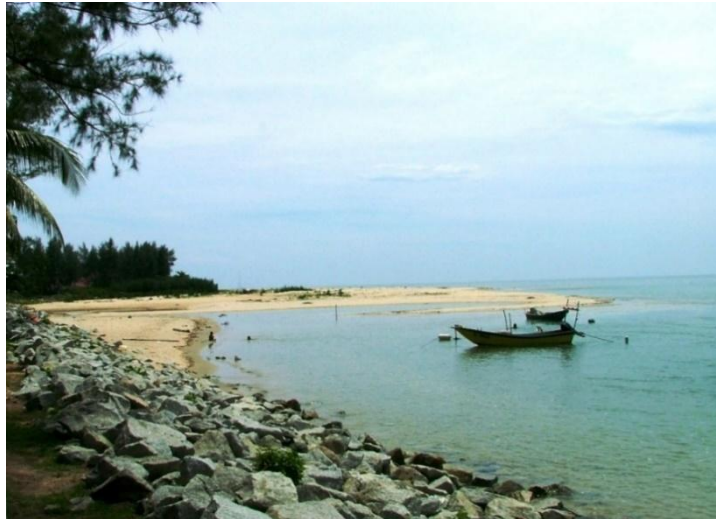
Figure 6: Coastal erosion at Pantai Kuala Ibai.
